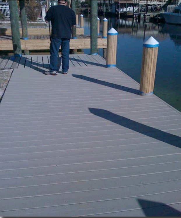
UDF-21 is applied to a wooden dock using a roller. One kit covers approximately 400 square feet (2 coats required).
