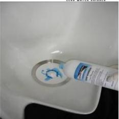
Pour about 30 oz. of water over the Drain Insert. Then slowly pour the entire contents of the Odor Barrier onto the Drain Insert. Wipe clean. The ZeroFlush Urinal is now ready for use.
