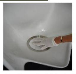
Press down on the drain insert until you feel and hear a slight popping sound. The insert must be tight.
