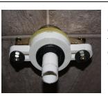
Remove old rubber gasket and Clean flange and drain Thoroughly. Install New flange Coupler rubber Gasket and tighten bolts.
