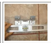
Install the wall bracket. Make sure the bracket is level and centered.
