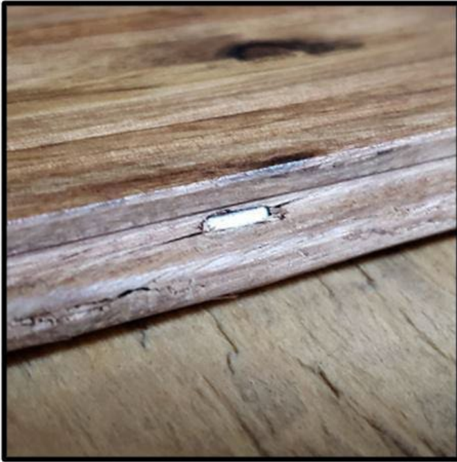
Cleat properly driven and no splitting
