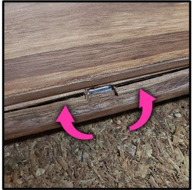
Cleat properly driven and some splitting
