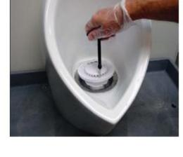
PULL UPWARD ON INSERT TO REMOVE.
